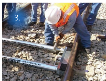
3. Inserting the MTW into the track and expanding the system via the threaded support poles
