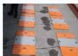
Installation of 700 x 430 x 35mm Light Duty Weigh Pads
