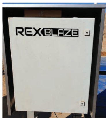
Weatherproof outdoor electrical cabinet
