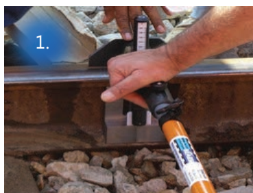
1. Measuring the height to determine packer size
